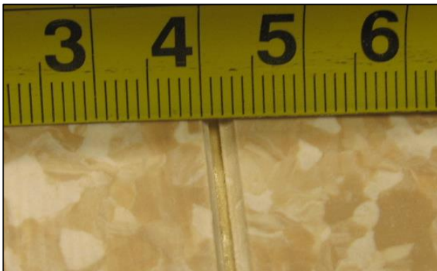
Maximum width of the groove - commercial flooring - 3.5mm / sport flooring - 4 mm
