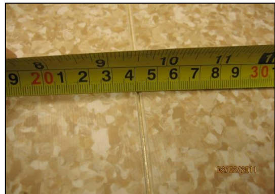
Maximum width of the groove - commercial flooring - 3.5mm / sport flooring - 4 mm
